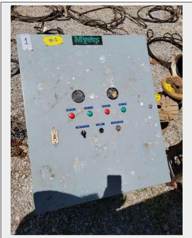
**Description**Myers lift station pump controller 3 phase 230v (needs control transformer)
